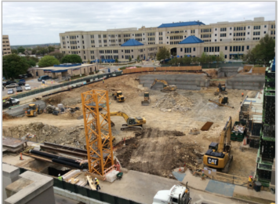
Excavation, Soil Retention, NT-ST Tunnel in Progress - 4/14/14
