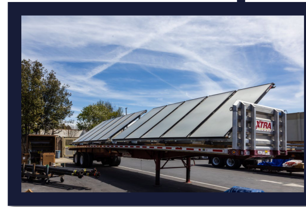
Shop fabrication and assembly
