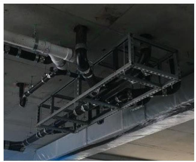
Sovent racks for the base of the system made installation of the most critical component very consistent between risers.
