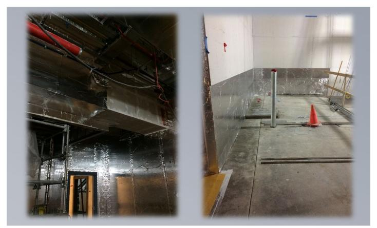
Radio Frequency (RF) Shielding
